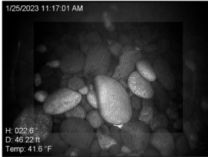
Figure 4: Survey Images of Stilling Basin Accumulation at Lower Granite Dam
