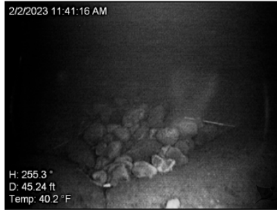
Figure 3: Survey Images of Stilling Basin Accumulation at Lower Monumental Dam
